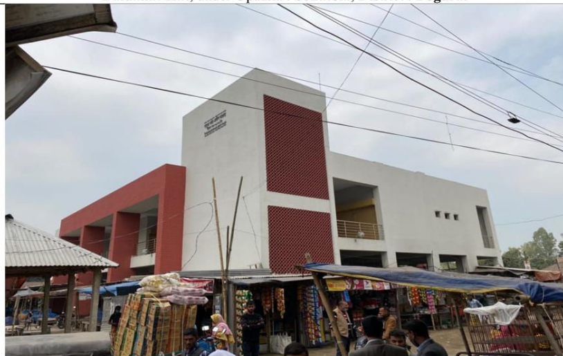
Baluahat Hat, under Upazila : Sonatola, District : Bogura.
