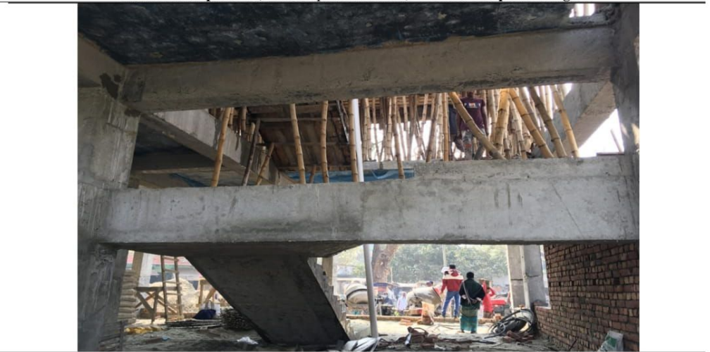
Ramchandropur Hat, under Upazila : Sadar, District : Chapainawabgan.
