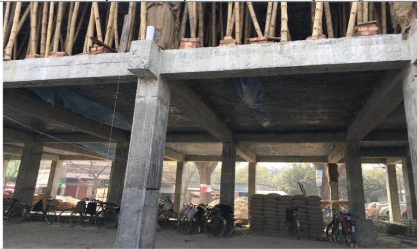
Ramchandropur Hat, under Upazila : Sadar, District : Chapainawabgan.
