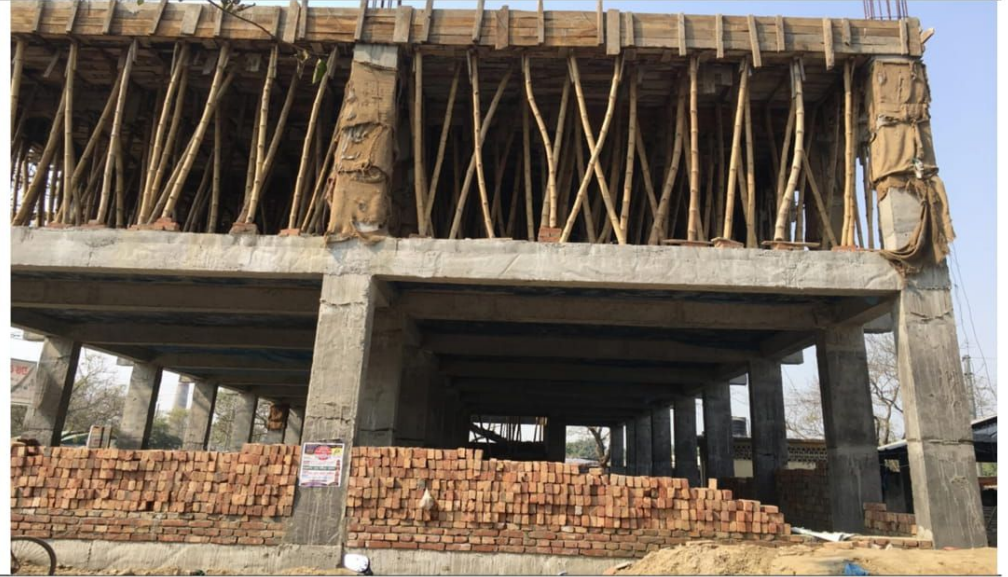
Ramchandropur Hat, under Upazila : Sadar, District : Chapainawabgan.
