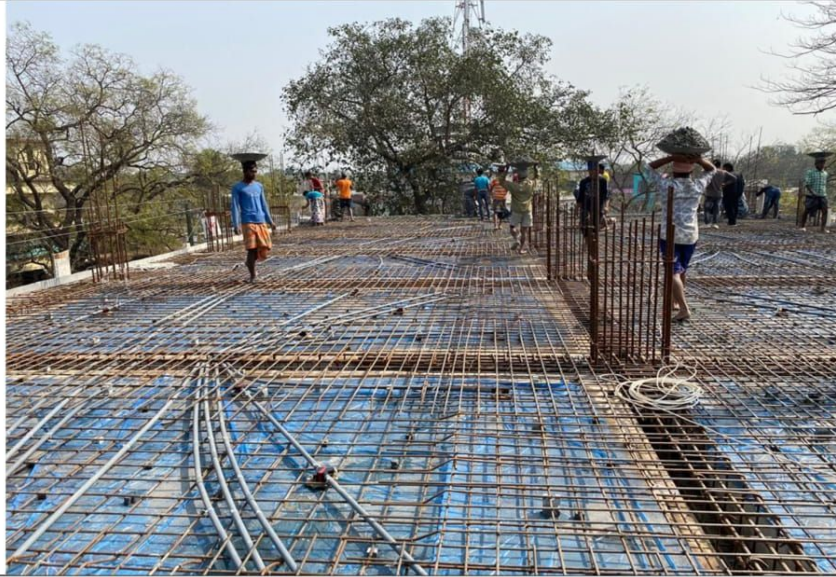
Ramchandropur Hat, under Upazila : Sadar, District : Chapainawabgan.
