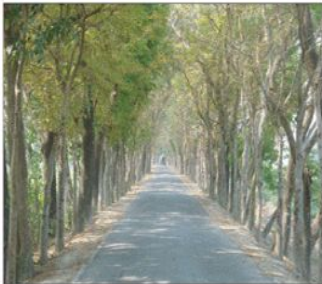
Bituminous Carpeting Road with plantation, Noakhali
