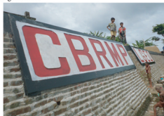
Village protection wall constructed with bricks that will protect the village houses from wave/flood action of the Haors, Tahirpur, Sunamganj.
