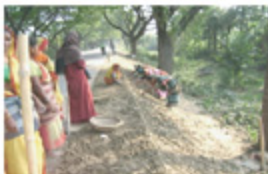
LCS women are carrying out routine maintenance works of the damaged paved road shoulder and slope.
