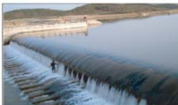
Mormermukh rubber dam on Shilock canal, Rangunia, Chittagong
