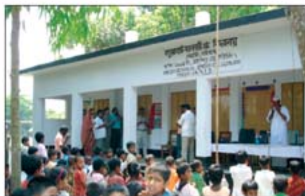
Kachuahaat Government Primary School Shaghatta Upazila, Gaibandha.
