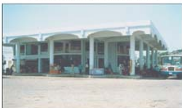
Narail Pura Bus Terminal
