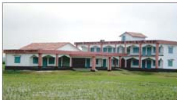
Dhunot Union Parishad Complex Building, Dhunot, Bogra
