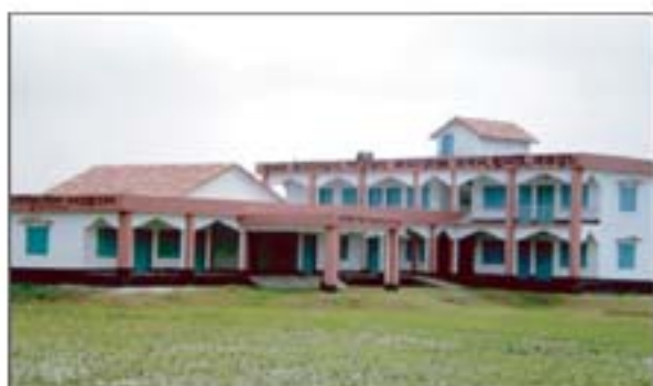
Dhunot Union Parishad Complex Building, Dhunot, Bogra
