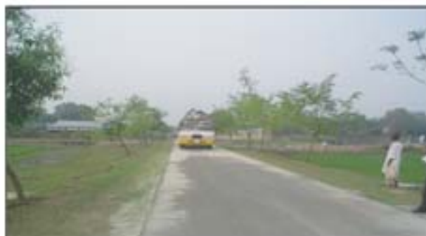
Road on maintenance in Mymensingh district.
