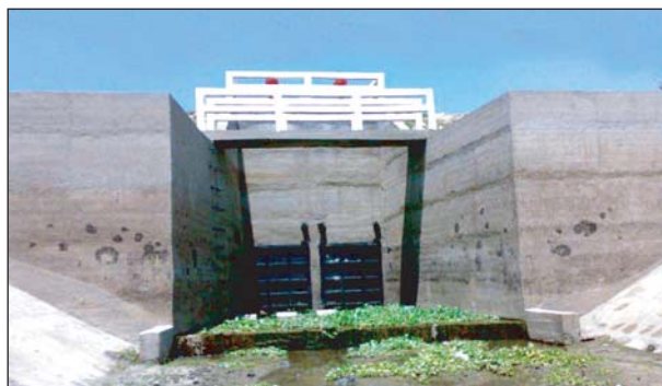
Photograph-18 : One two-vent regulator across Umed Ali Canal, Mirzapur, Tangail.
