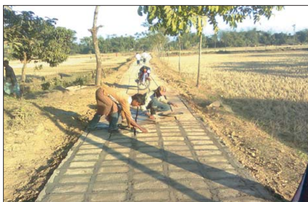
Photograph-44: Road being constructed with concrete block to help the communities in Sunamganj district under the Community Based Resource Management Project.
