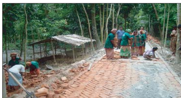
Photograph-50: A LCS group constructing HBB road
