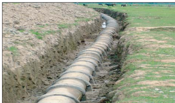
Photograph-19 : Buried pipe constructed under Joygaon-Painda irrigation sub-project, Sunamgong
