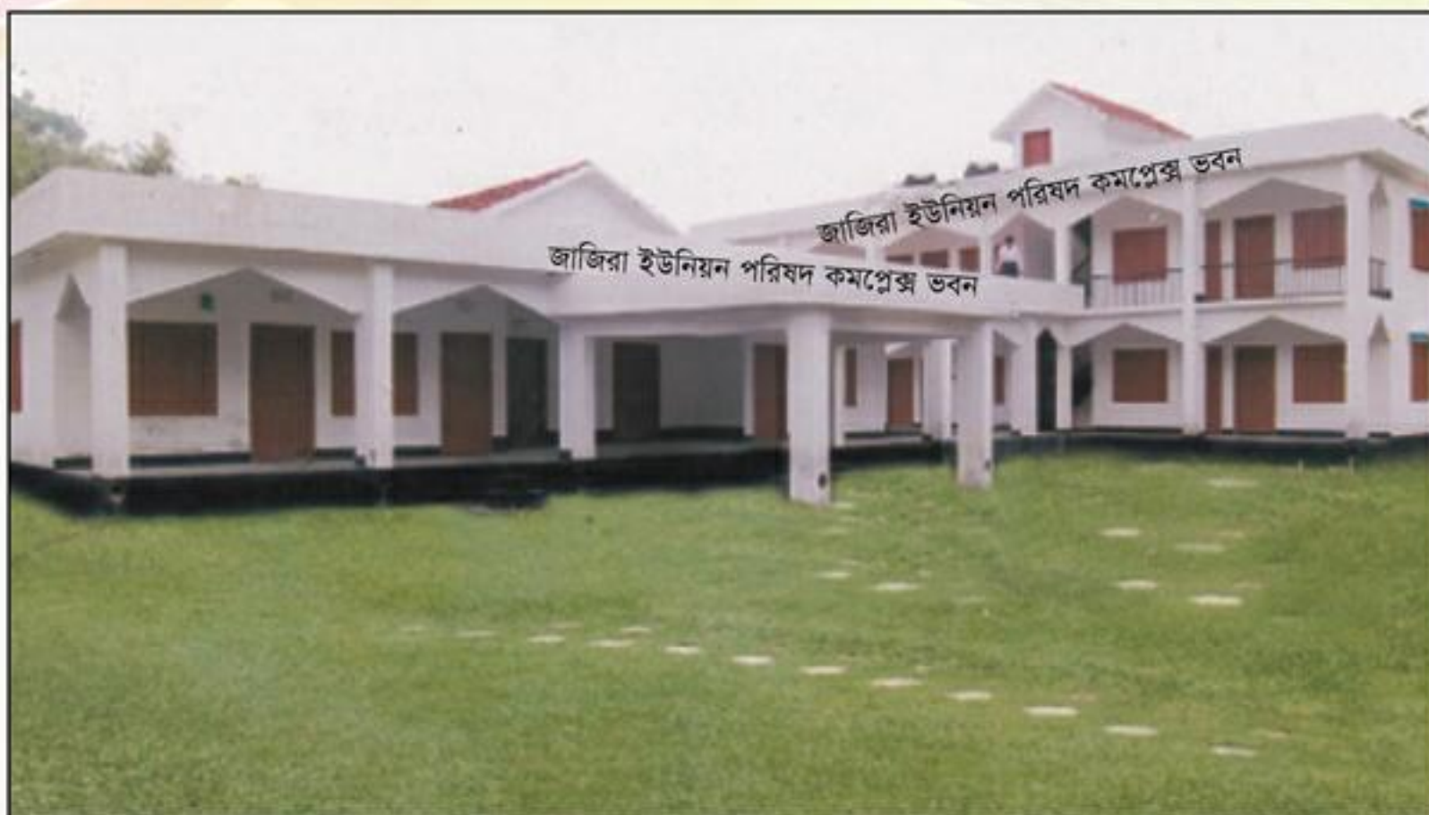
Janjira Union Parishad Complex Building, Shariatpur.
