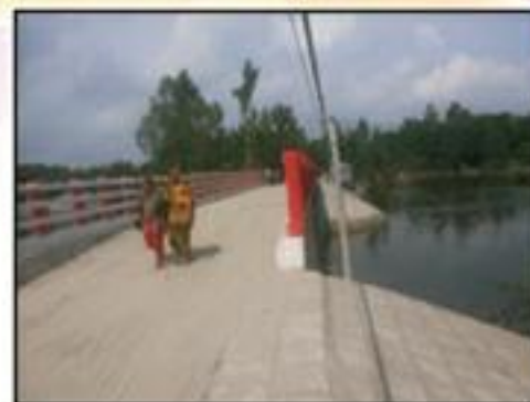
Bridge construction in Kurigram
