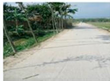
Upazila road constructed in the Haor region
