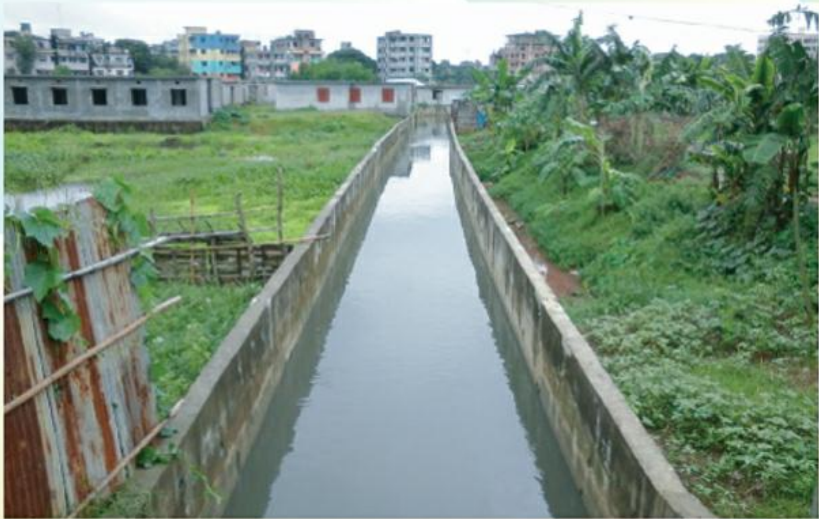
Under Construction drain in Gazipur City Corporation
