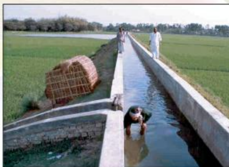
Agrani sub-project irrigation canal, Sadar, Chapai Nawabganj
