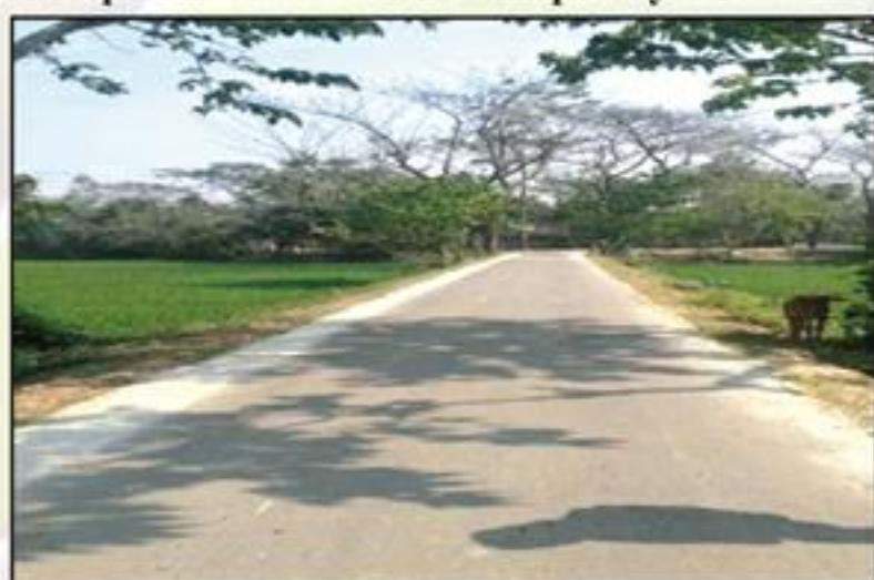
Dakhsin bazaar-Khalpar Ayabari pool road, Begumganj, Noakhali.
