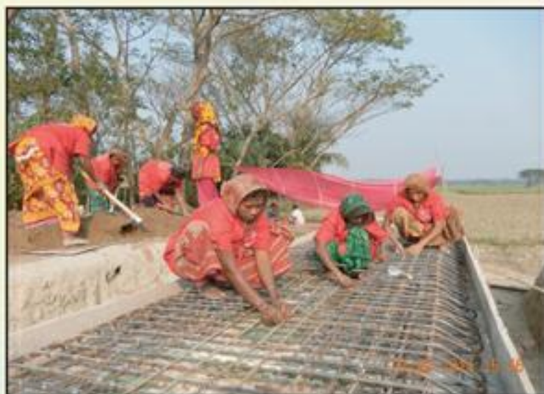
U-drain construction by LCS women
