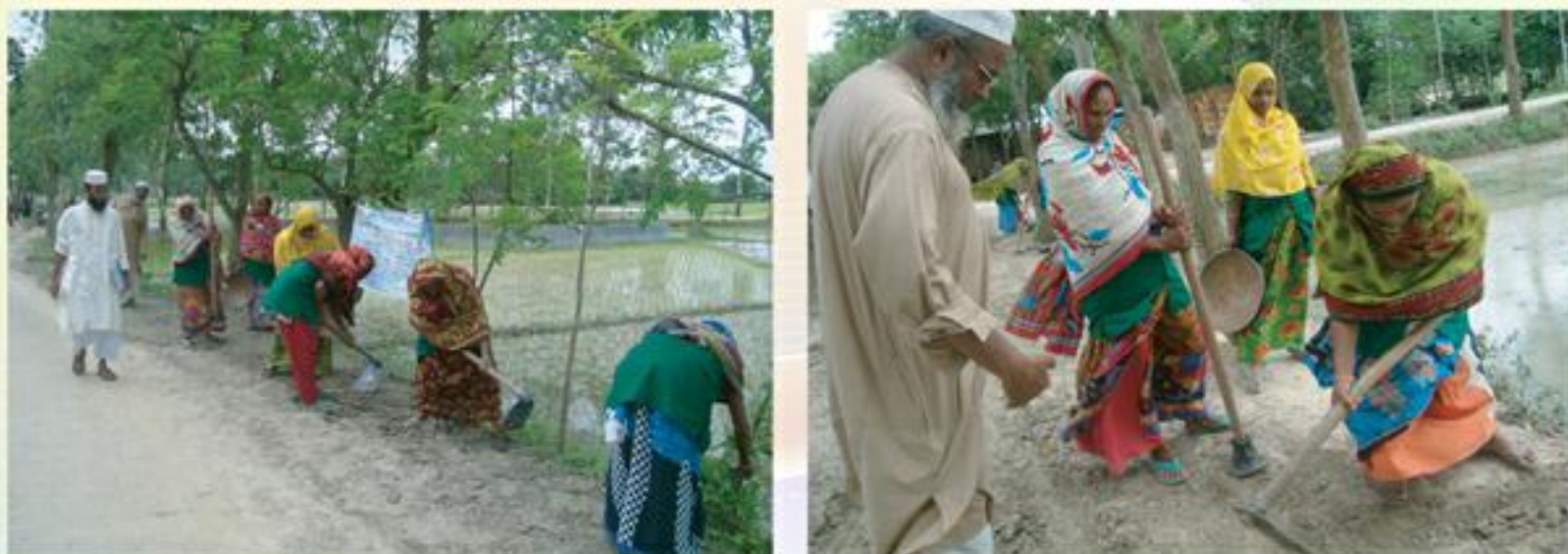
Maintenance job by RERMP-2 workers
