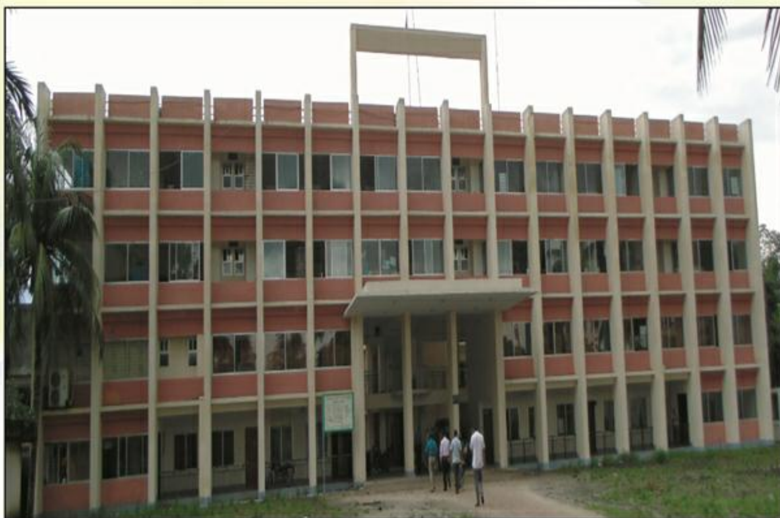
Upazila Parishad Building, Kotalipara, Gopalganj
