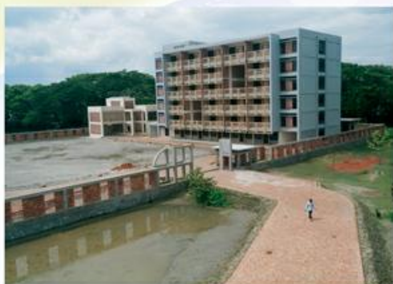
PTI hostel building, Jhalokathi
