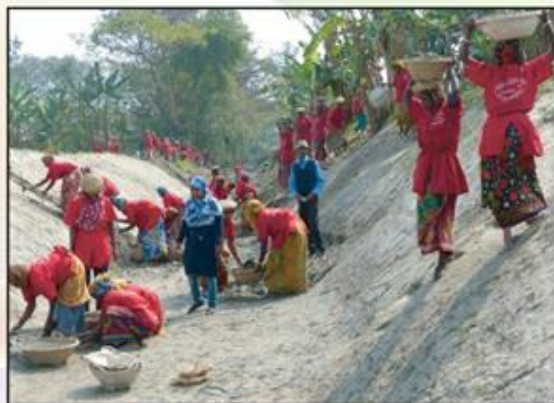
Canal excavation by LCS women
