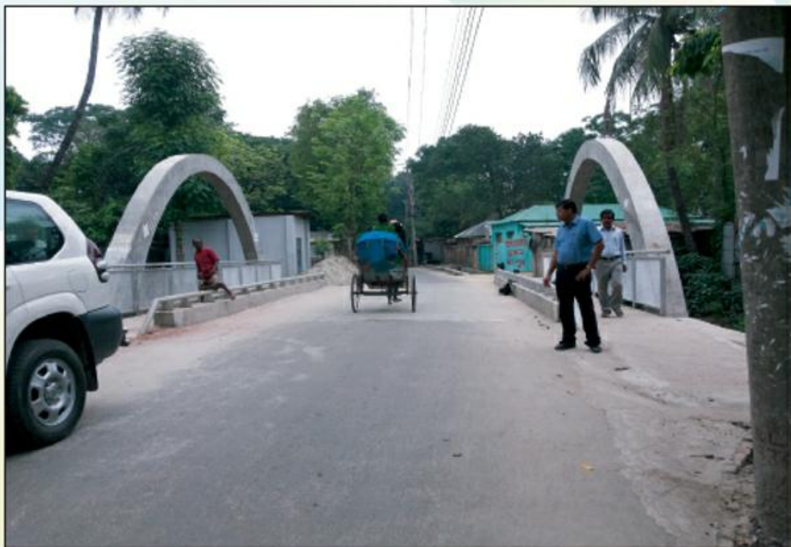
A bridge constructed over Shama Sundari Canal.
