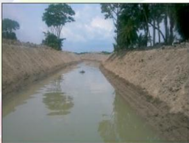
Re-excavation of canal under sub-project at Auliarchar, Kalkini under Madaripur
