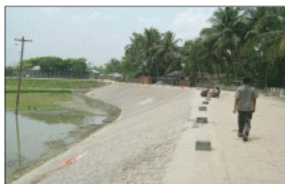
Placing of blocks to protect Pourashava road from erosion
