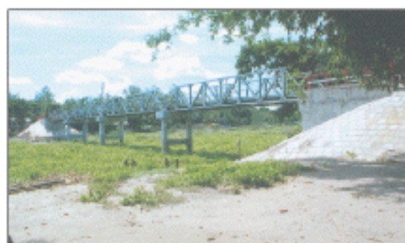
One 80 m long portable steel bridge on the Panchasarutia RHD - Randhumbari Road, Sadar, Sirajganj
