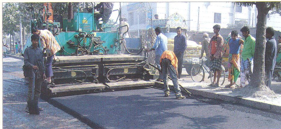
Bituminous carpeting work is in progress on Bangabadhu Road under Narayanganj Paurashava being implemented by LGED's UGIIP.
