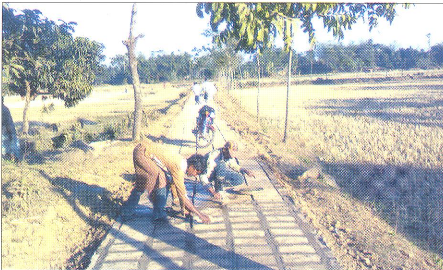
A concrete block road constructed by CBRMP.
