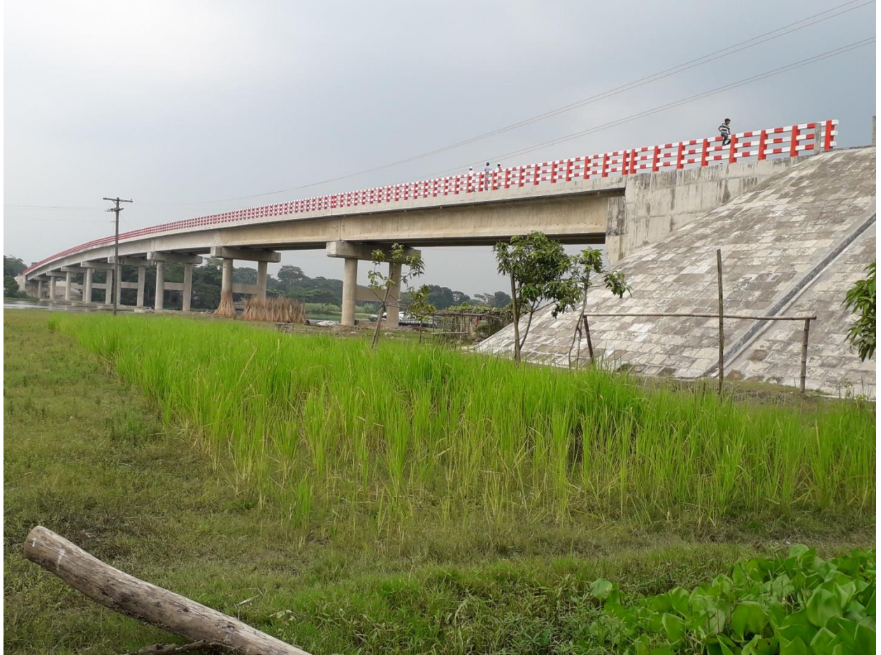
306.40 m long Joynagar Bridge at Zajira, Shariatpur
