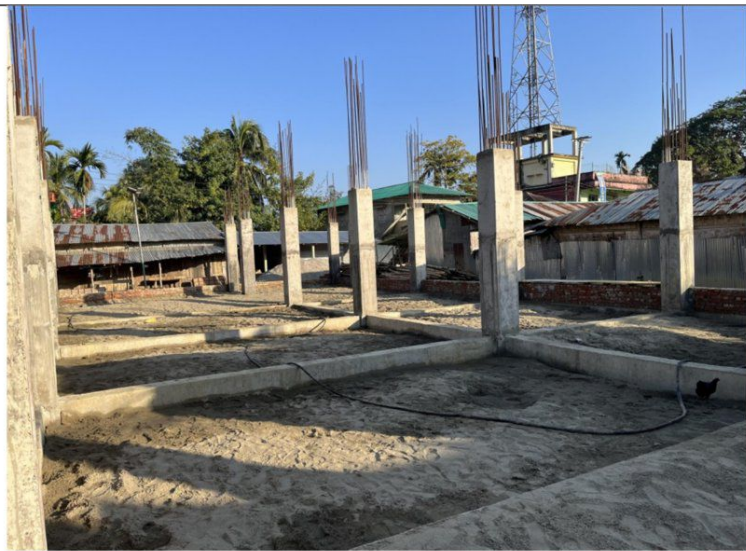
Refarpara Bazar, under Upazila : Alikadam, District : Bandarban.
