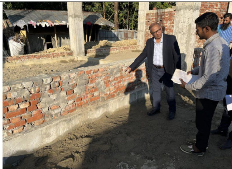
Refarpara Bazar, under Upazila : Alikadam, District : Bandarban.
