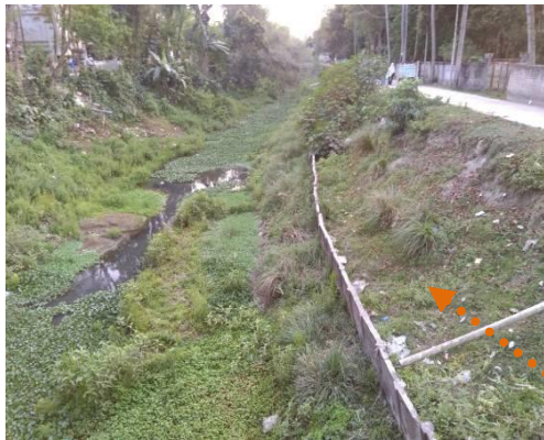
Canal banks need slope protection
