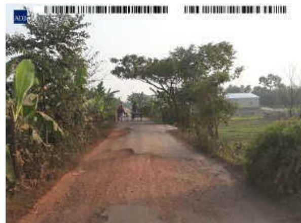
Condition of existing BC road surface at chainage 3000
