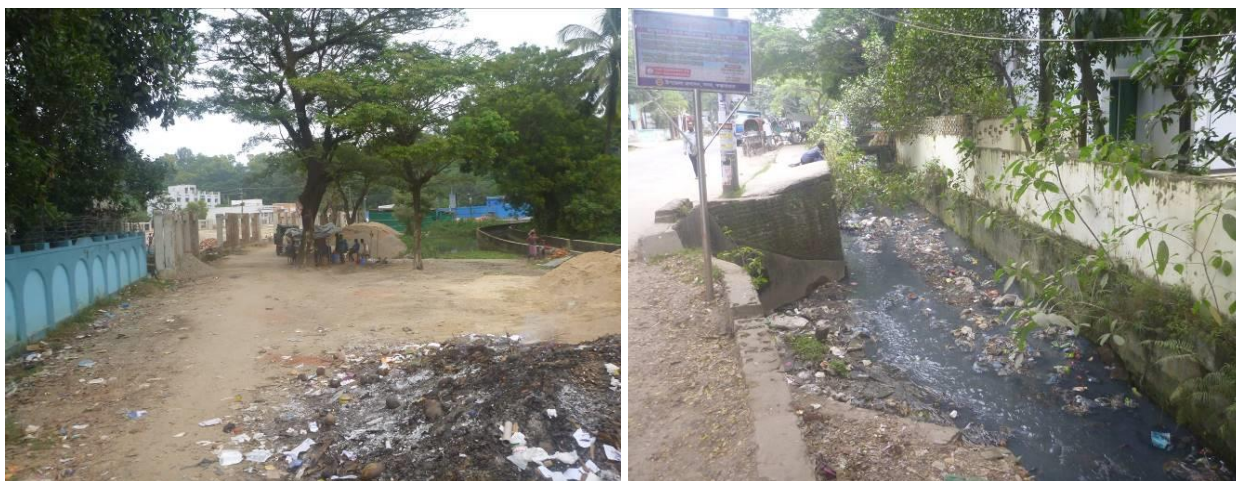
Photographs 2.2.1 (b): Current Situation of the Outfall
