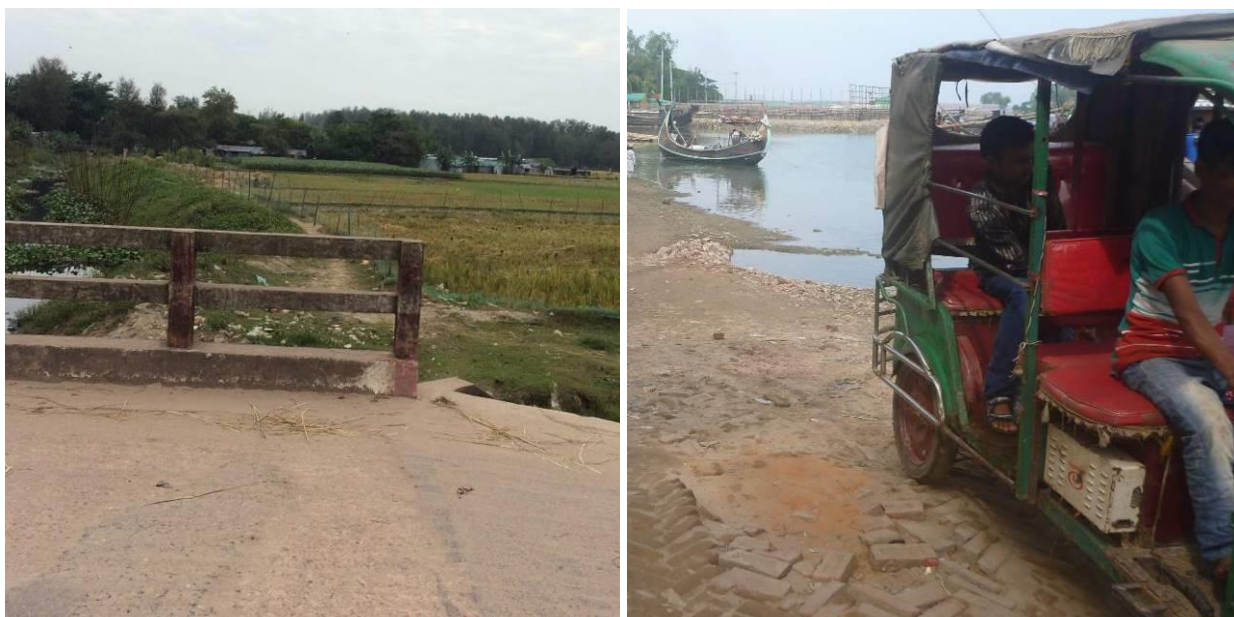
Photographs 2.2.1 (b): Current Situation of the Outfall
