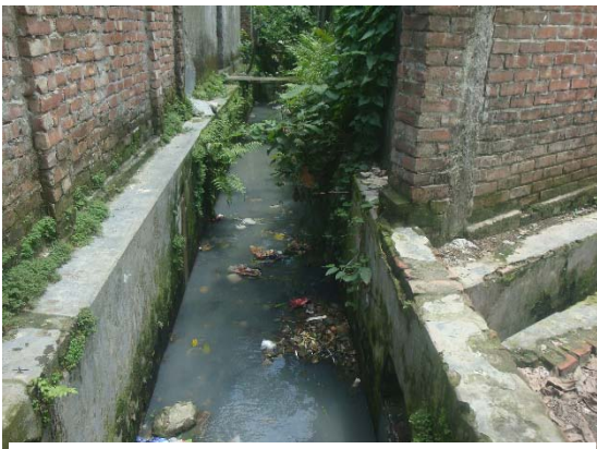
Figure 1 Open out faff need cover slab at kharampotti road
