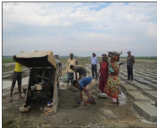
Construction of palestineblock at Gagrajore under Borkapon union.
