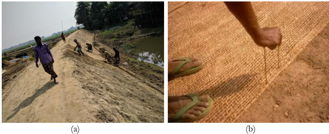
Figure 4.10: Photographs of (a) Slope Preparation by LCS; and (b) JGT Placement on Prepared Slope
