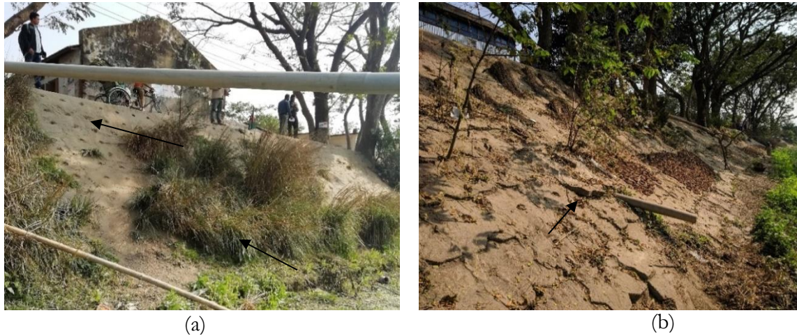
Figure 3.7: Photographs of (a) Slope Condition at 14 th January 2019; and (b) Loosened CC Blocks along Slope
