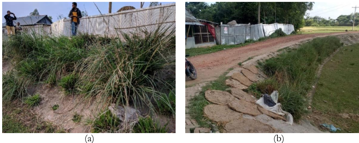
Figure 3.10: (a) Slope Condition of the Paschimbag, Azmiriganj, Habiganj after Facing Two Monsoons; and (b) Slope Condition of the Site after Facing Three Monsoons
