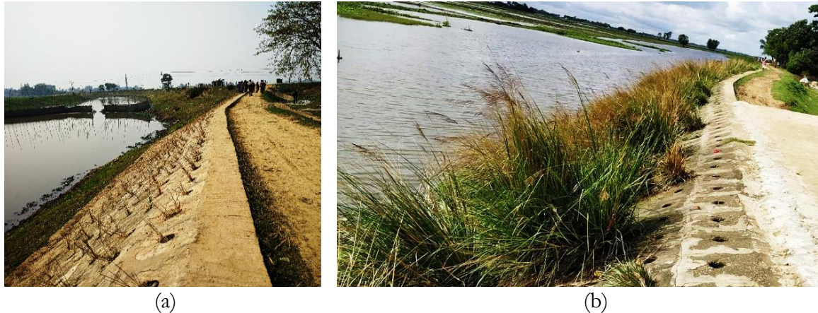
Figure 3.14: Photographs of Slope Condition at Vatipara, Baniachong, Habiganj: (a) 24 Days after Plantation; and (b) After Facing One Flood
