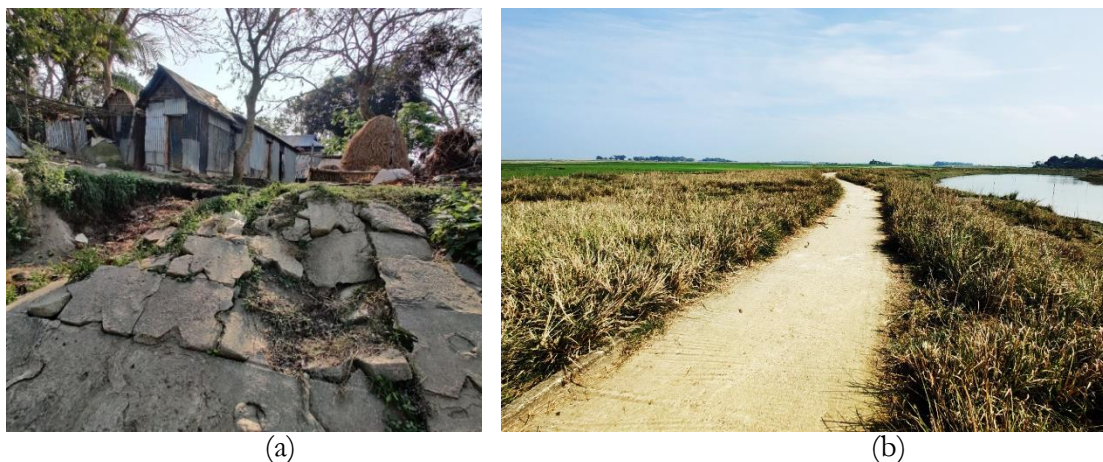
Figure 3.15: (a) Broken Slope by Sealed Block; and (b) Vetiver Source at Hayatpur, Khaliajuri, Netrkona
