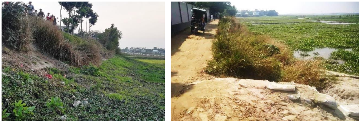
Figure 3.8: (a) Slope Condition after Facing Two Monsoons; and (b) Slope Condition after Facing Three Monsoons
