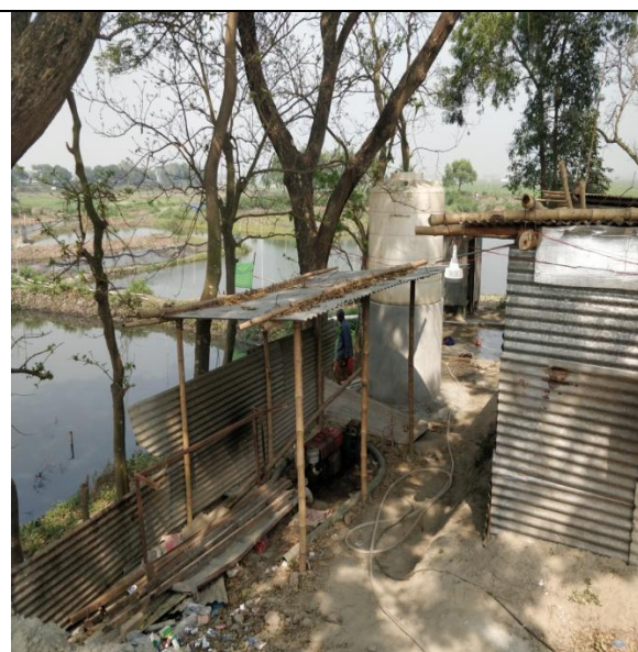
Water supply and sanitation facility point are close to each other (not recommended) and difficult to access
