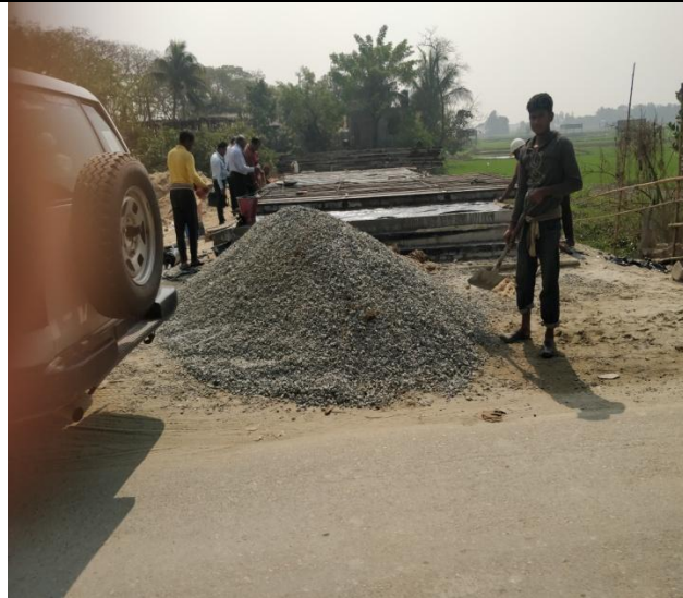
Stockpiling construction materials (stone chips) and curing micro compaction piles at the road side (not desirable)
