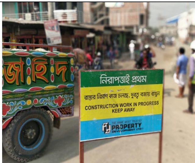
Non-specified warning sign posted at the wrong place (junction point of three roads)
