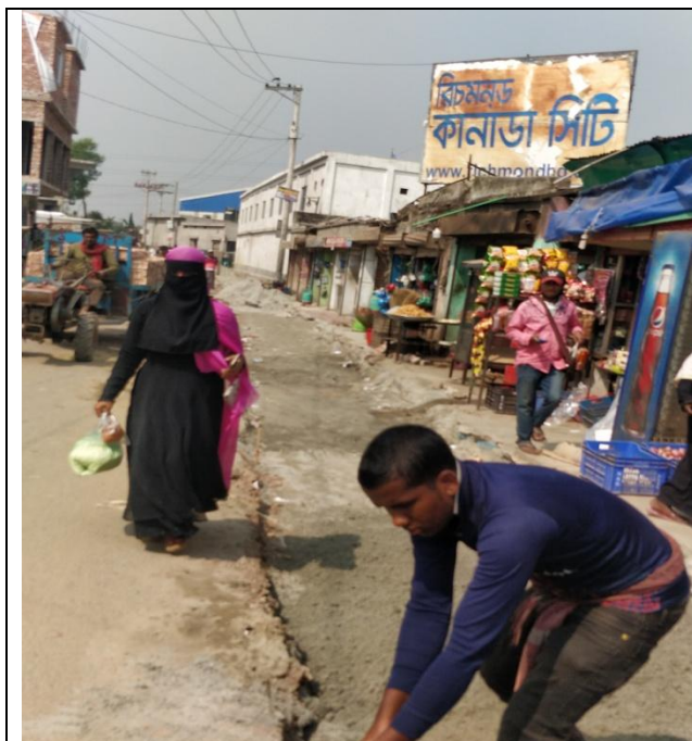
No safety barrier alongside the vertical cut and fill of the road under improvement
