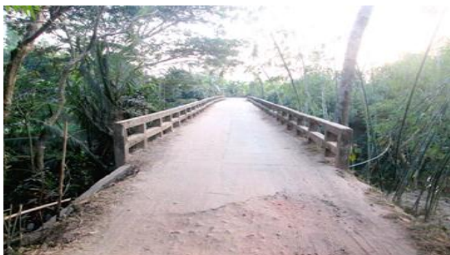
Present condition of 45.00m Long RCC Girder Bridge at Moricha GC - Naikhongchari GC via Paglir bill Natunpara road (Ukhiya Part) in Ukhiya Upazila of Cox's Bazar District (W9.3)
