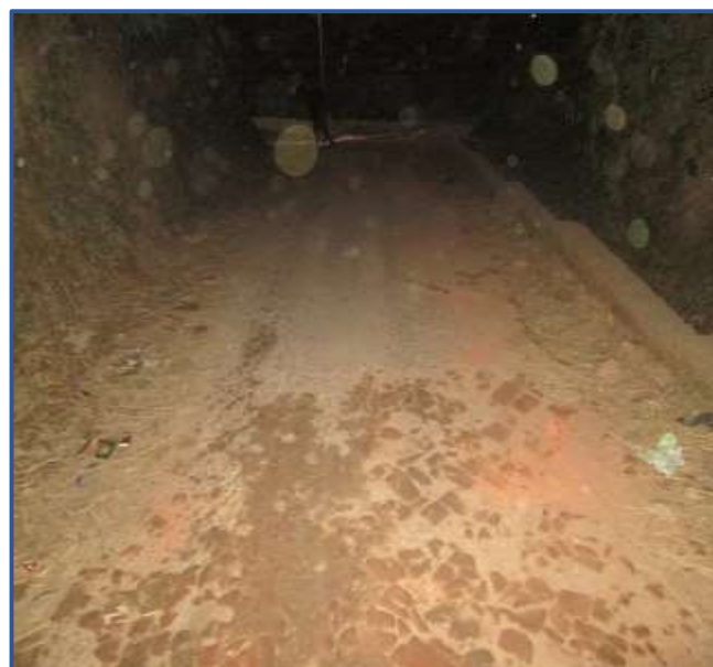
Some parts of the road having BC upper layer and some parts BFS
