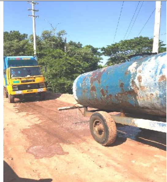
CRDP-2/LGED/Savar/NCB/2018/W-04 Dust control by watering road under construction
