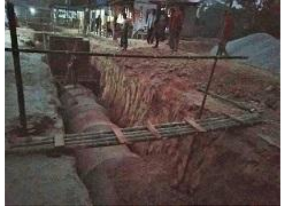
CRDP-2/LGED/GCC/NCB/2018/W-01 Temporary Crossover facility at pipe laying site
