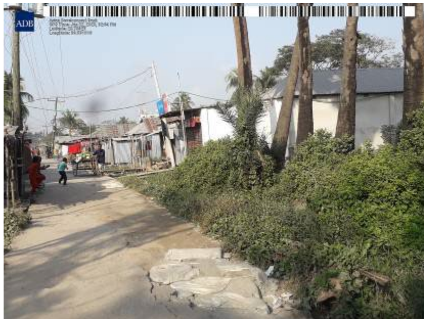
Existing road condition of road at chainage 650
