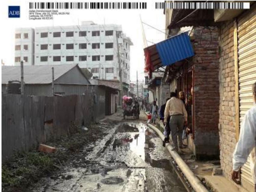
Photo at chainage 400
