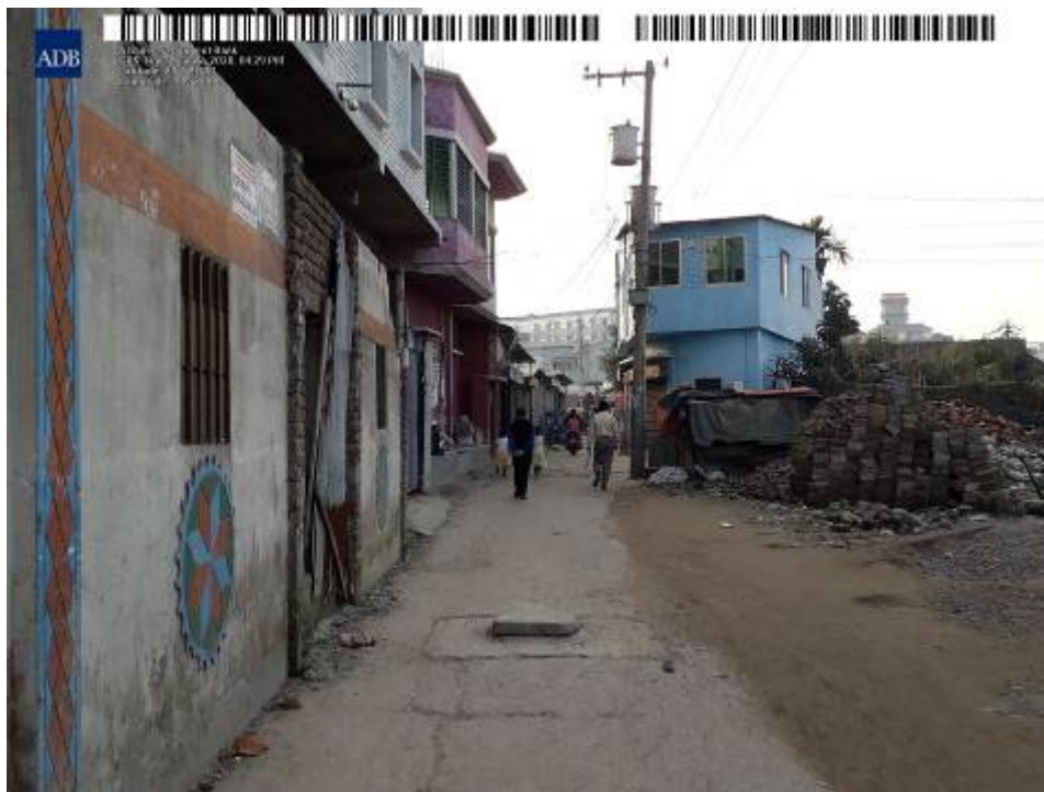
Existing road condition of road at chainage 475
