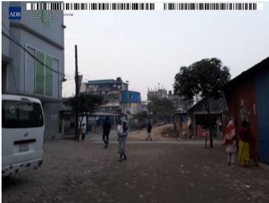
Figure 2: Photograph of existing condition of Road from Dighiborabo Abu Sayed Market to Jatramura Canal
