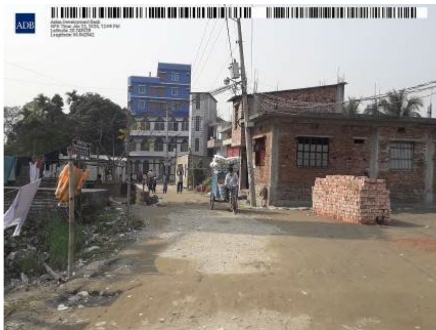
Existing drainage condition at chainage 550
