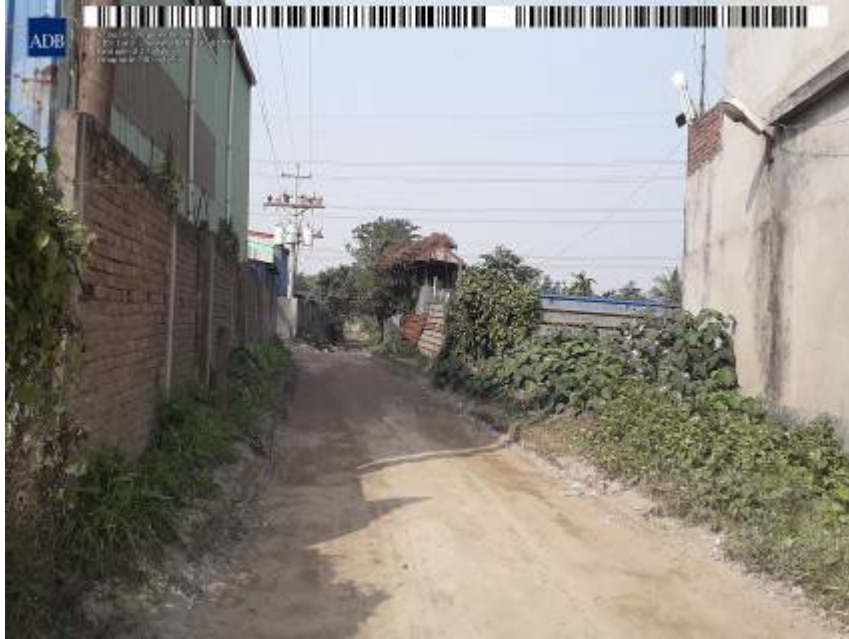
Photo at chainage 125
