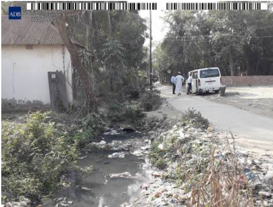
Existing drainage condition at chainage 875
