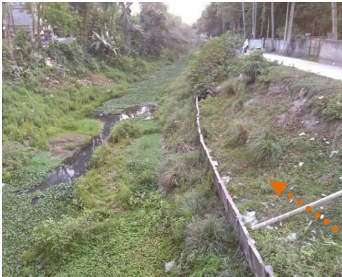
Canal banks need slope protection
