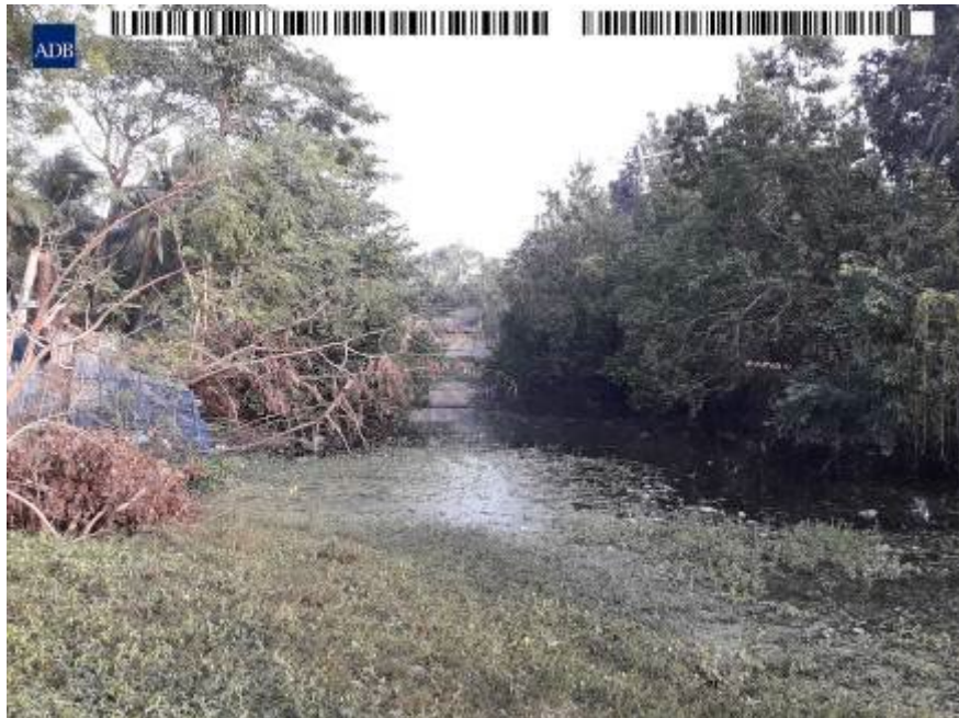
Existing condition of the canal at chainage 300
