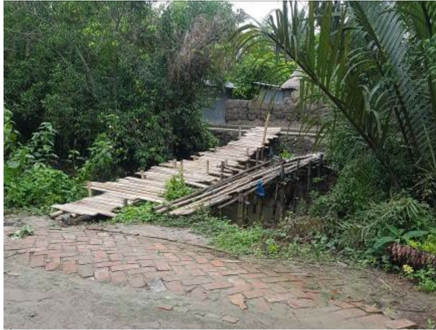
Existing condition of the bridge construction location
