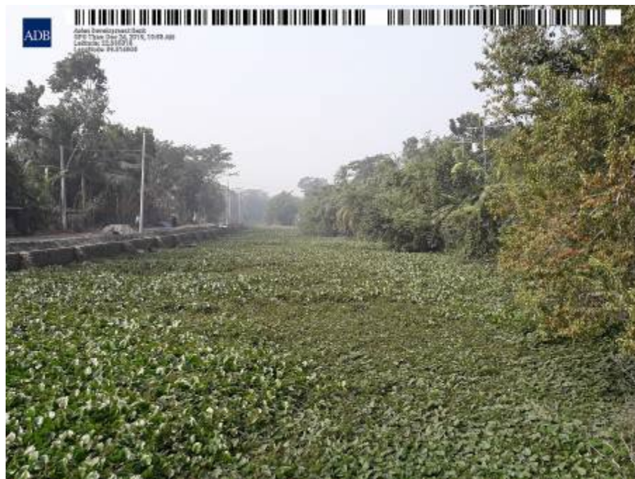
Existing condition of canal at chainage 560
