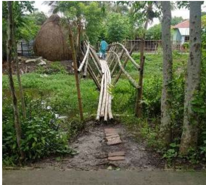
Photo of the bridge construction site
