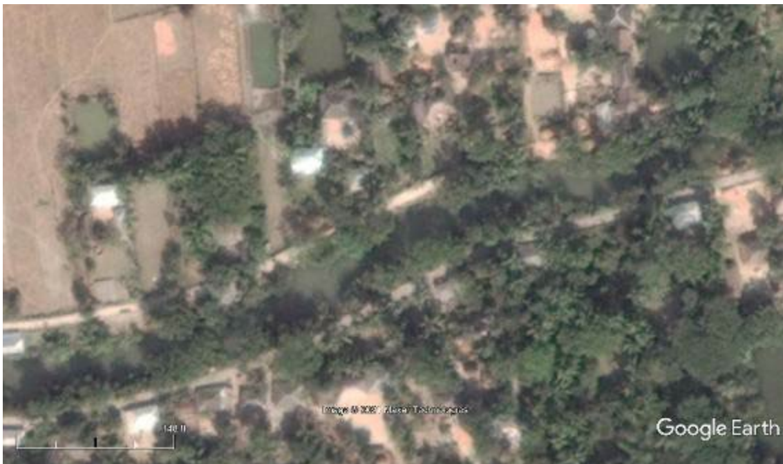
Google Earth Image of the bridge construction site
