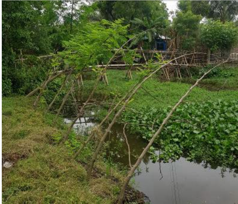
Existing condition of the bridge construction location
