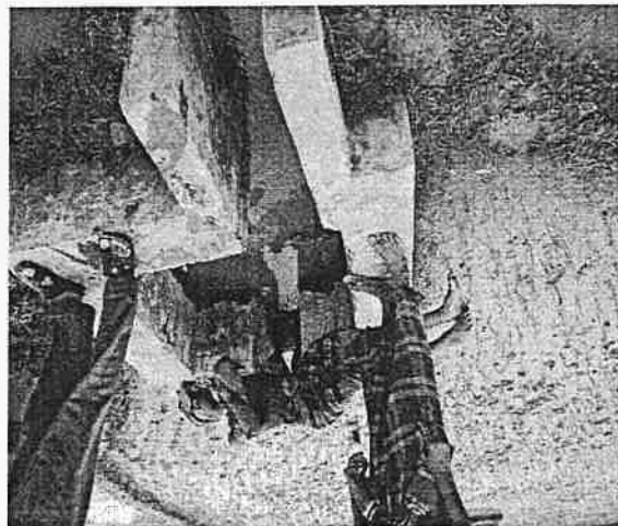
Standpipe airtvent which is not sufficiently high and venting water SP 33096 Saherber Gaon, Sunamganj
