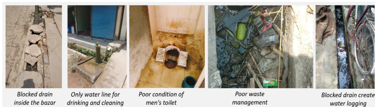
Figure 6-9: Current status of infrastructure
