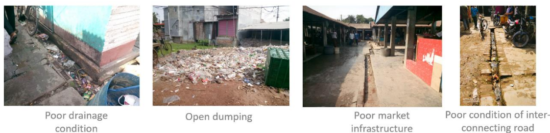
Figure 7-6: Poor Sewerage and waste management
