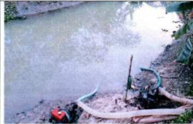
A view of drawing water from the canal at East Sonakhali Subproject, Amtali, Barguna
