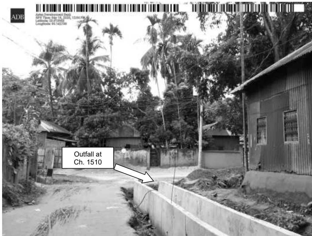
Figure 7: Photograph of the outfall of the Box drain from Singair College to Singair Old Bus Stand from Ch.500m to Ch.1510m
