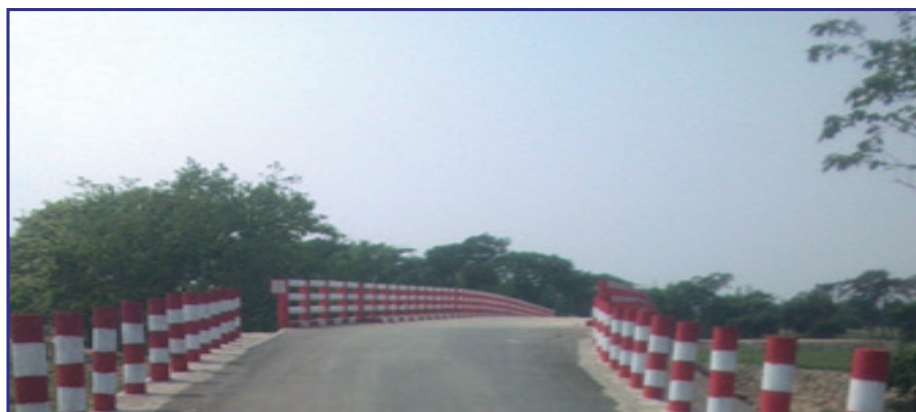
28m span pre-stressed concrete girder bridge over Gumai River
