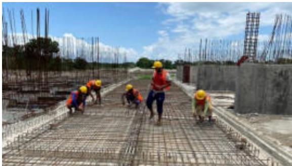
Compost plant rod binding and shuttering works, Soula, KCC W-01
