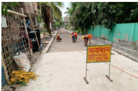
RCC road pavement from Ch: 606 to 665m on Taher more to Kawratola road M.S rod binding, Mongla W-01
