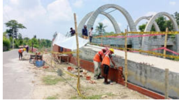
Approach ramp brickwork in Chalna W-01
