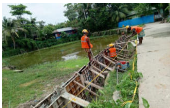
RCC Palisading casting from Ch.634 to 645m besides Taher more road, Mongla W-01
