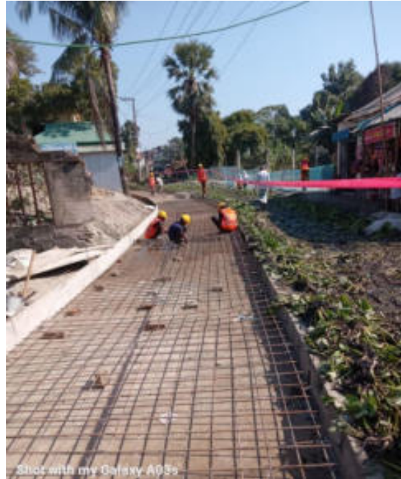
Shahalam - bari road, RCC road rebar binding work ongoing on GCC - W03,
