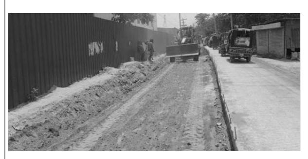
Continuous vehicle movement provision by constructing alternative strips at Porshi GC To Murapara GC Via Rupganj Road, Package Ruphanj W-04
