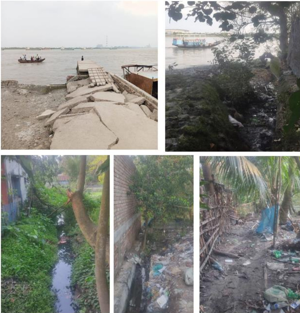
Drainage outfall and current condition of the drains of Chana Pourashava
