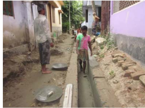
Labours are working without any PPE.(PDP-35)
