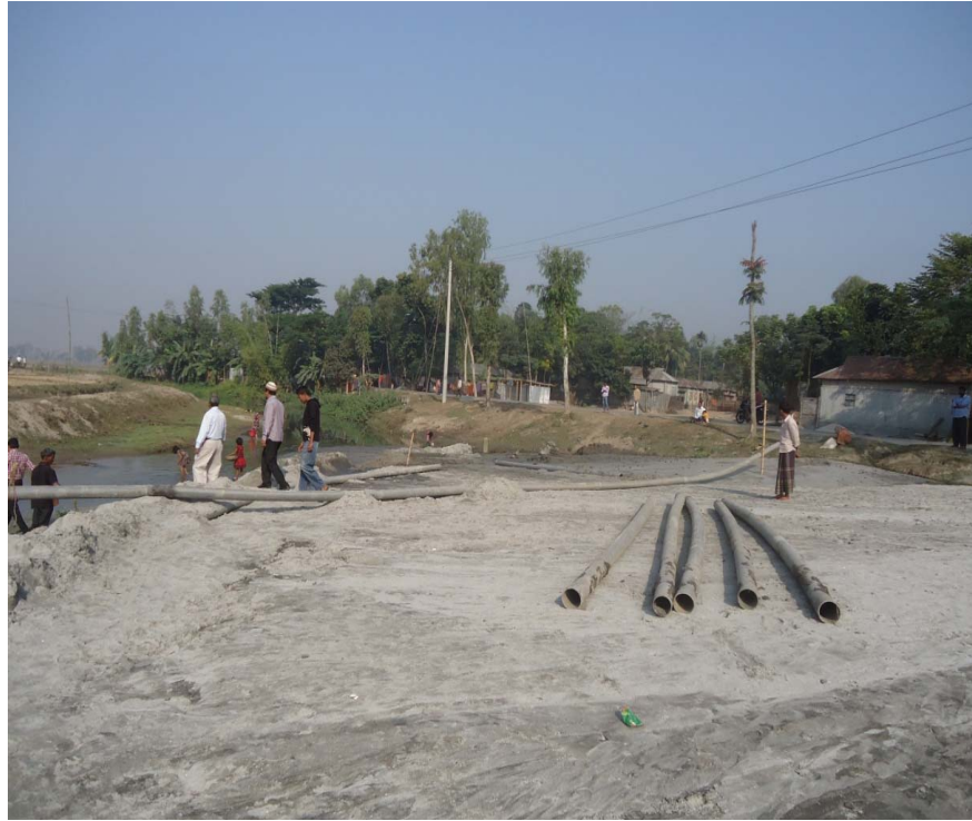
Ongoing filling of the proposed site for bus terminal
