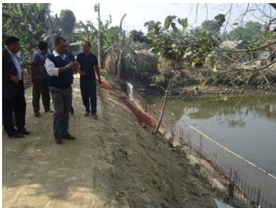
Construction of new palasidings
