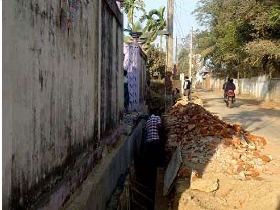
Ongoing construction of drain at Ghosgoun Madrasha Road (Non use of PPEs by Workers)
