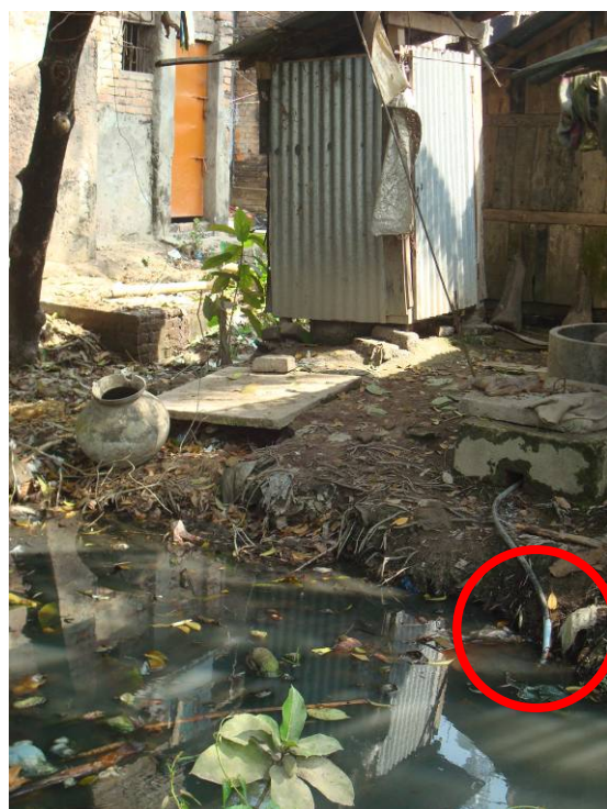
Plate 4.1: Constructed as a sanitary toilet but connected with canal
