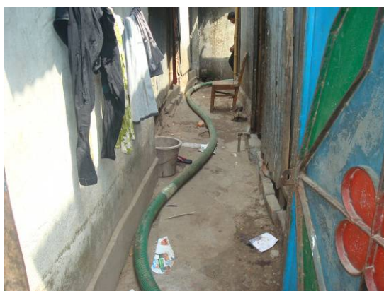
Plate A3: 100 meter pipe being stretched from the vaccutug to the pit latrine
