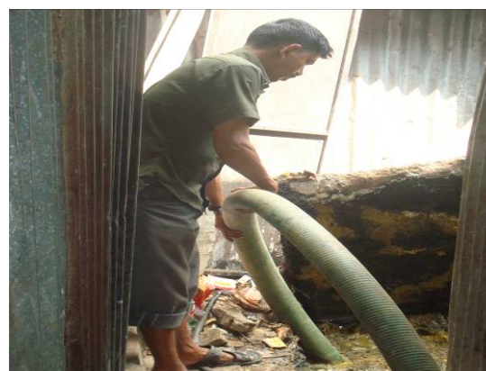
Plate A4: Sludge is being collected from a pit latrine
