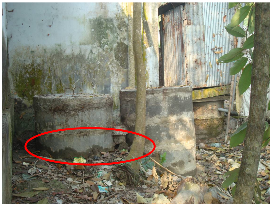
Plate 4.1: There is Leakage in the Ring – So the Latrine is no Longer Hygienic
