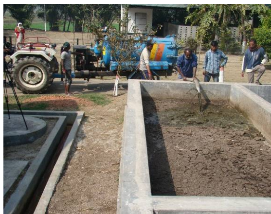
Plate A10: Collected faecal sludge emptied in the drying bed of co-composting plant at Baradi, Kushtia
