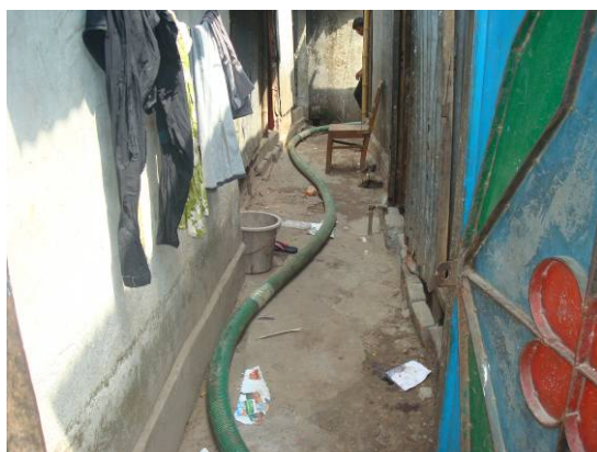
Plate A3: 100 meter pipe being stretched from the vaccutug to the pit latrine
