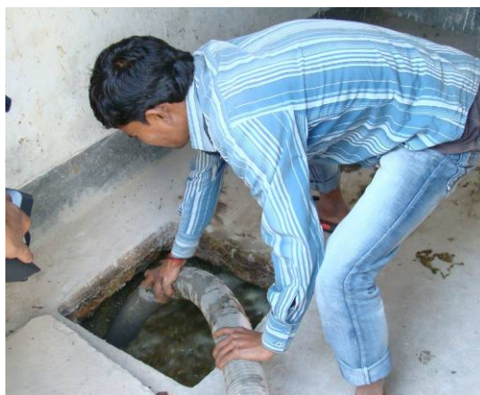
Plate A9: Septic tank located inside the household premise being emptied with vaccutug.
