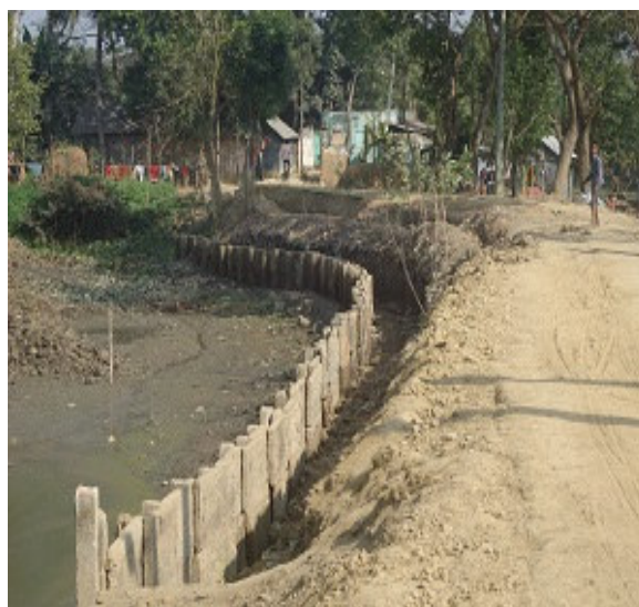
Construction of new palasiding at Madhabpur
