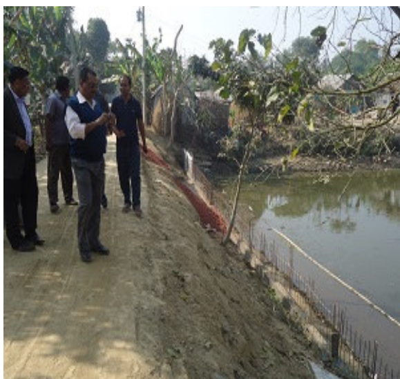
Construction of new palasiding at Madhabpur
