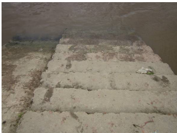
Kalardoba Boat Landing Facility (Zila Boud)* Ghats are mainly Concrete Step type.
