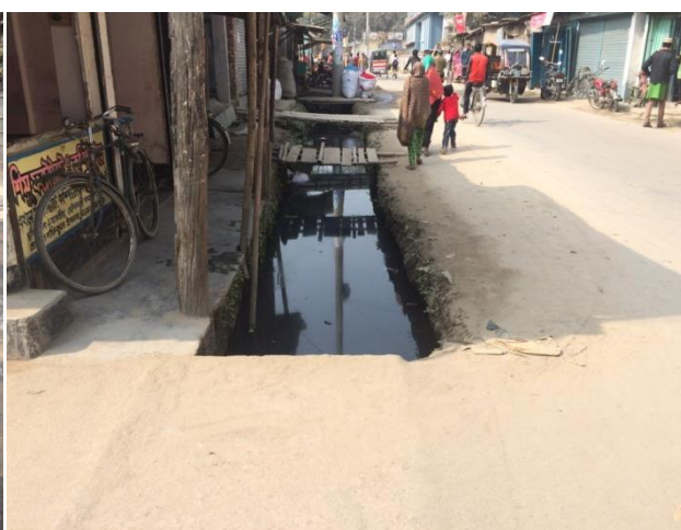
Temporary access over drain to the shops at Lalmonirhat
