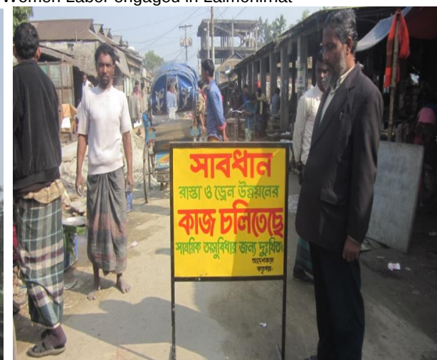
Safety Sign at Muktagacha
