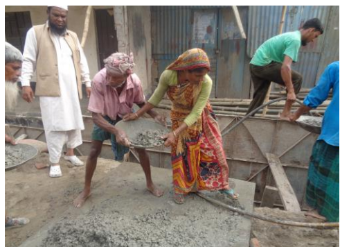
Women laborer in construction work: Bera PS
