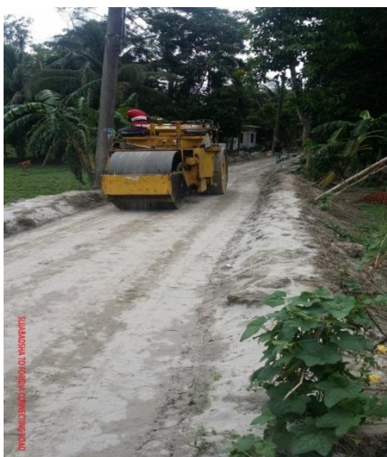
Road: Laxmipur Pourashava
