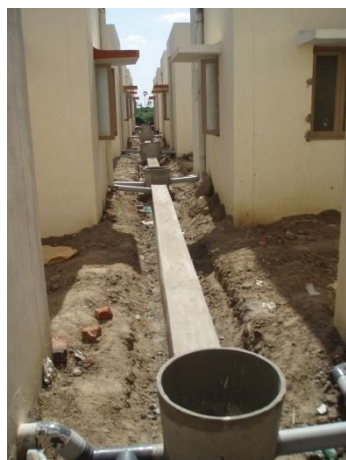
Figure 0.7 Shallow sewer system at Tsunami affected colony, Tamil property boundaries, hence the need for the community to agree to the arrangement.
