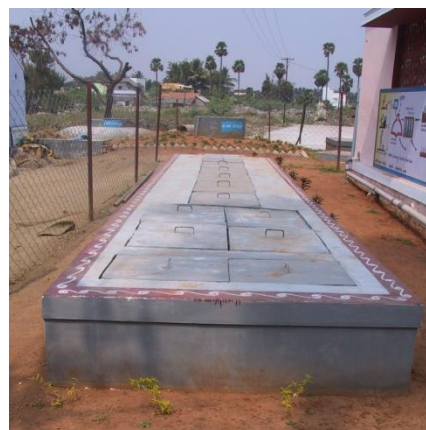
Figure 0.3 – Improved septic tank for public toilet, Tamil Nadu, India
