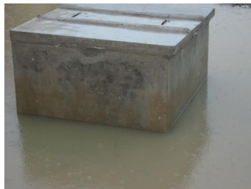
Figure 0.4 – Water tight improved septic tank
