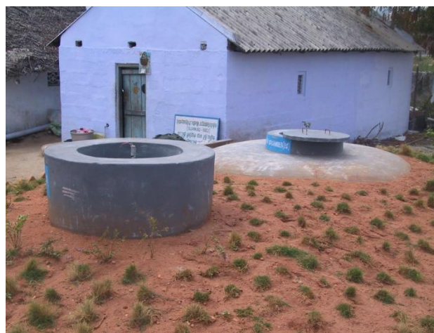
Figure 0.5 – Fixed dome biogas digester
