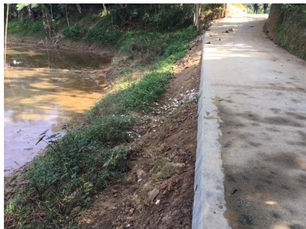
Rangamati: Sadhona Road to Buddhist Community Area: RCC Road and example of incomplete road verge works (29 Nov 2016)
