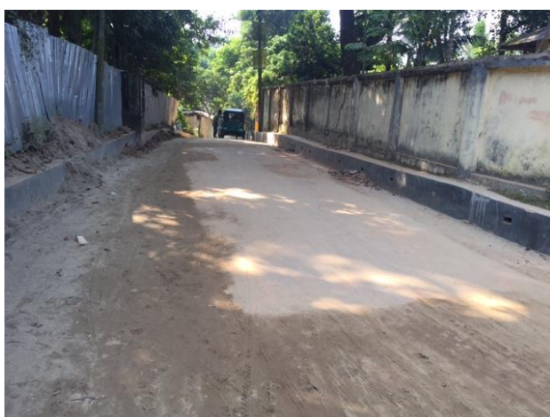
Rangamati: Road 20 Rehabilitation: WBM sub-base rejected after Contractor was allowed to cover with sand (29 Nov 2016)
