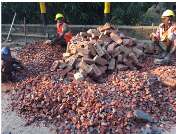
Bandarban: Manual production of Brick aggregate for WBM, photo (28 Nov 2016)
