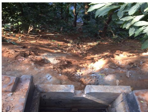
Rangamati: Bejoynagot Road to Bano-Behere connection: RCC Road and example of incomplete drainage outfall (29 Nov 2016)
