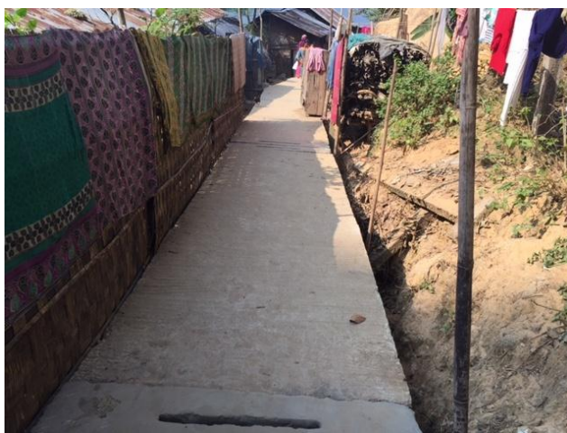
Rangamati: Completed RCC covered drain with footpath, at Haji-Sarker Road in Muslim Community (29 Nov 2016)
