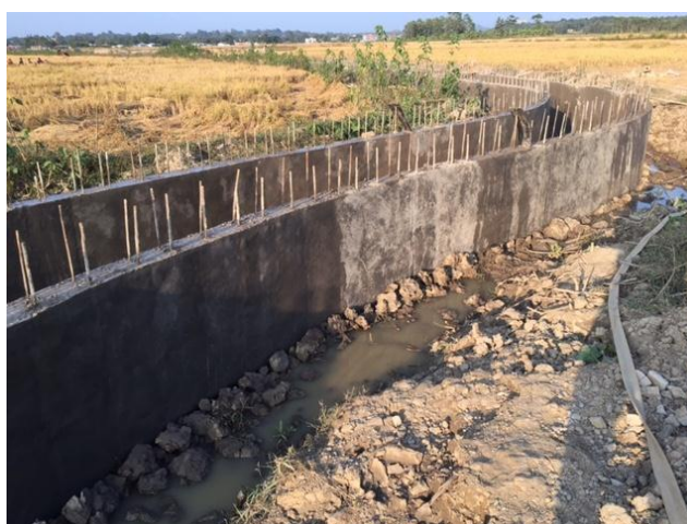
Khagrachari: RCC outfall drain at Anandanagar Area – (30 Nov 2016)
