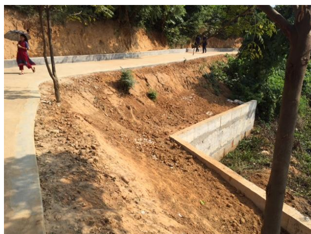
Rangamati: Bejoynagot Road to Bano-Behere connection: RCC Road and example of side filling and road verge. (29 Nov 2016)
