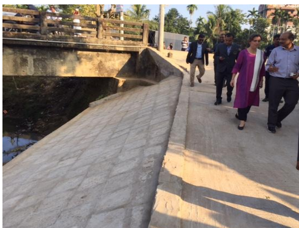
Khagrachari: RCC Rehabilitation of Pankphaiyapara Road - Safety barrier/ Handrail protection be considered along road verges where a fall hazard is a concern (29 Nov 2016)
