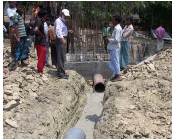
Steel pipe with flange to connect to uPVC pipe SP33059 Baneswardi, Faridpur
