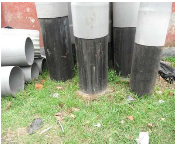
Factory made connection between flanged steel and uPVC pipes SP 41008 Goshinga, Gazipur
