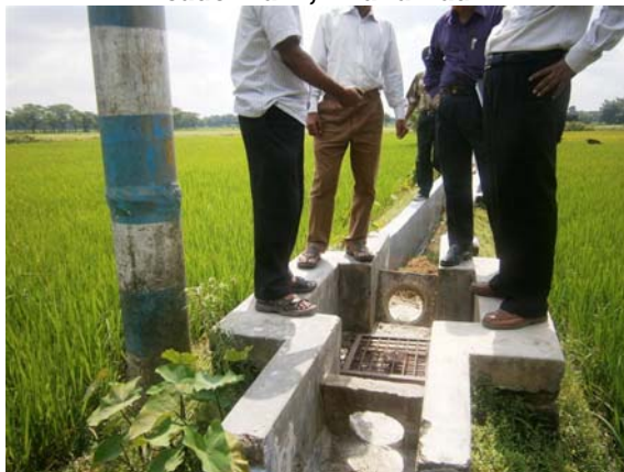
Air vent Standpipe & Outlet Box, Kharia Nadi
