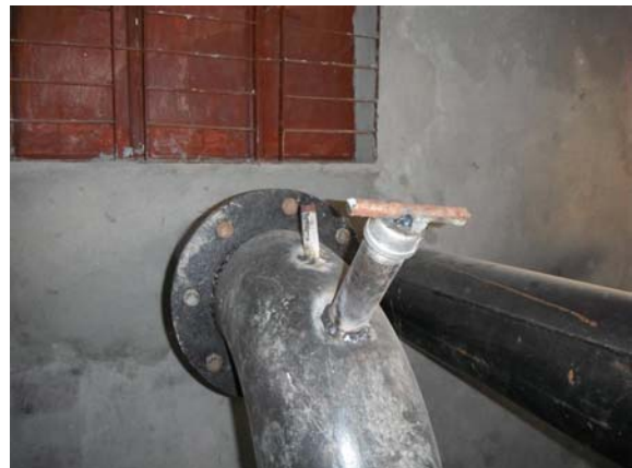
1½ inch pipe fitted to 8 inch outlet pipe to allow pump priming. ½ inch pipe also fitted for draw off of cooling water for diesel engine
