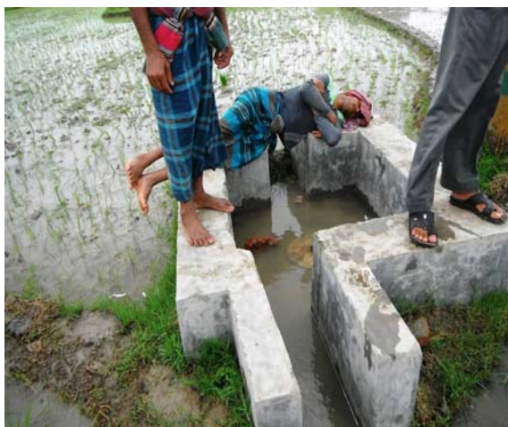
Outlet riser box with alfalfa valve for flow control SP 25288 Dariapur, Chapai Nawabganj
