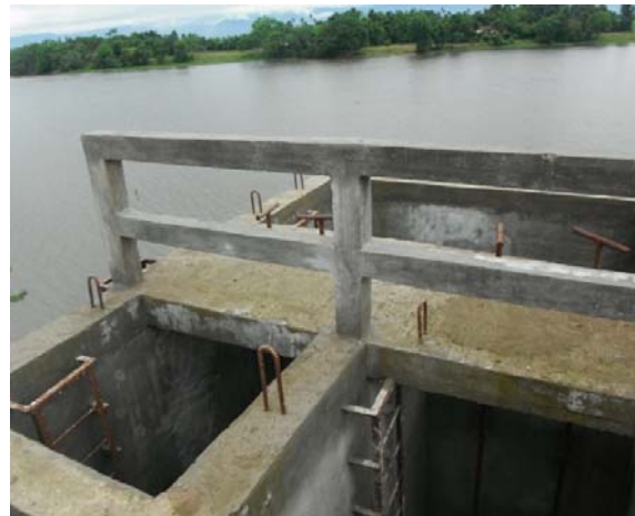
Operating Platform on top of Header Tank, SP 33096 Saherber Gaon, Sunamganj
