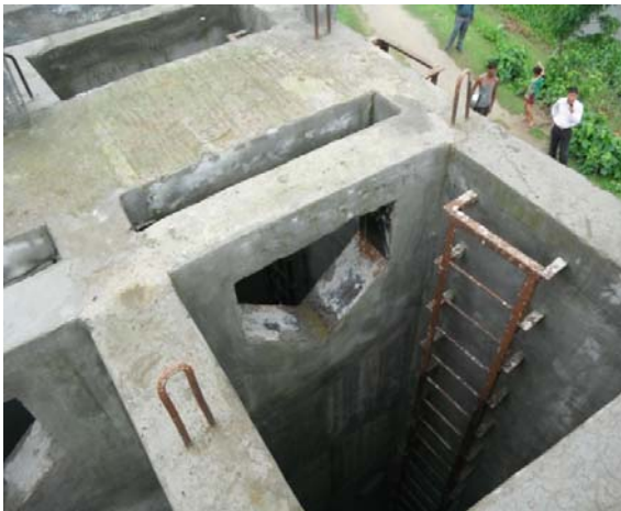
Flow measurement V-notch weir between compartments 2 & 3, SP 33096 Saherber Gaon, Sunamganj
