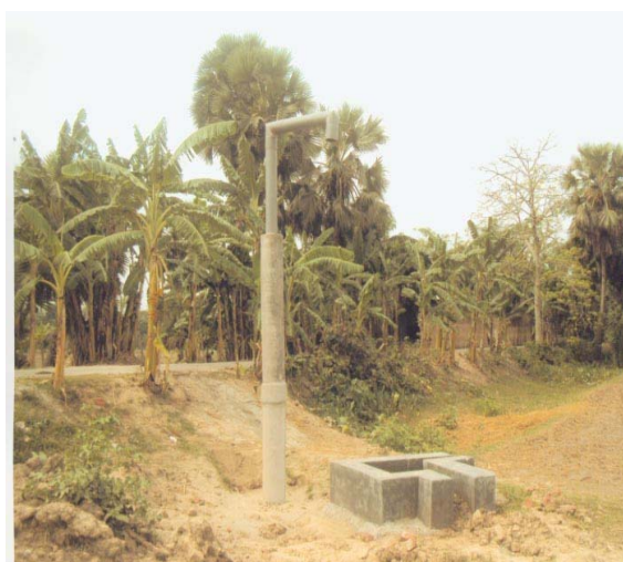
Airvent standpipe about 5 m high (near to head of system) SP 33044 Bajra Panai, Faridpur
