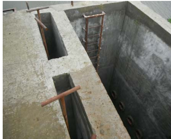
Handles to open / close valves from top of tank, SP 33096 Saherber Gaon, Sunamganj
