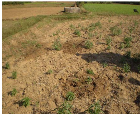
Leakage from joints of buried concrete pipeline
