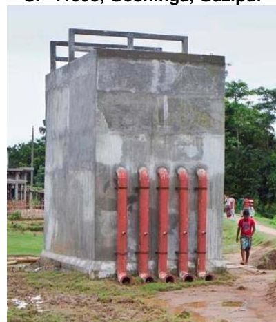
Completed Header Tank SP 33096 Saherber Gaon, Sunamganj
