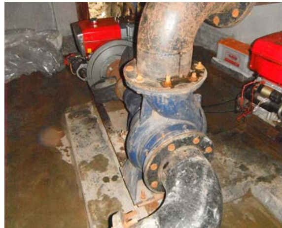
Diesel Pump set arrangement Banewardi Pump House
