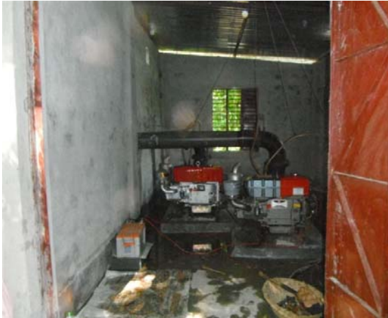
2 diesel motors & pumps installed in pump house, SP33059 Banewardi, Faridpur
