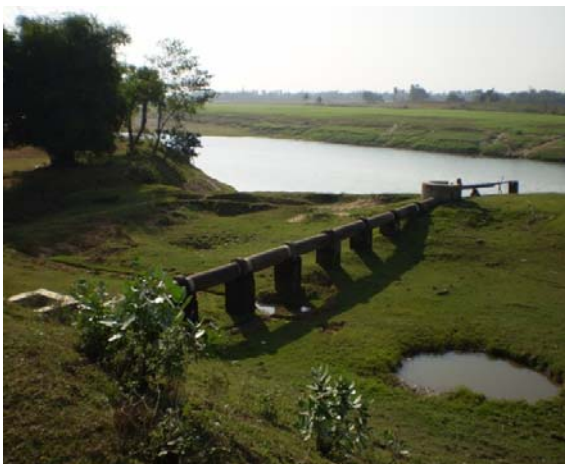
Elevated concrete pipe aqueduct (Orissa, India)
