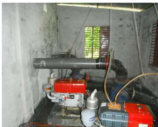
Two pump sets with Type F Milner Pumps, and diesel engines with rated outputs of 28 and 32 BHP, Banaswardi, May 2014
