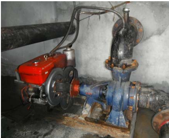
Diesel Pump set arrangement Banewardi Pump House
