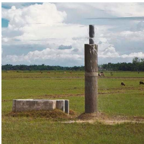
Standpipe airvent which is not sufficiently high and venting water SP 33096 Saherber Gaon, Sunamganj
