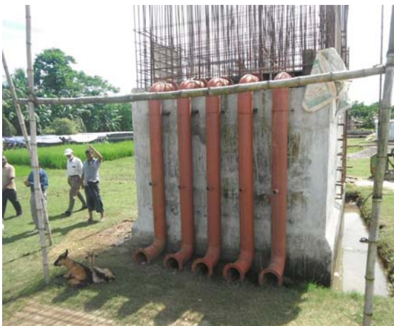
Header Tank under construction SP 33096 Saherber Gaon, Sunamganj
