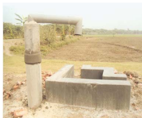
Airvent standpipe about 1.4 m high (at tail of system) SP 33044 Bajra Panai, Faridpur
