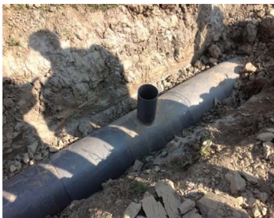
T-shaped on pipe for airvent standpipe SP33059 Baneswardi, Faridpur
