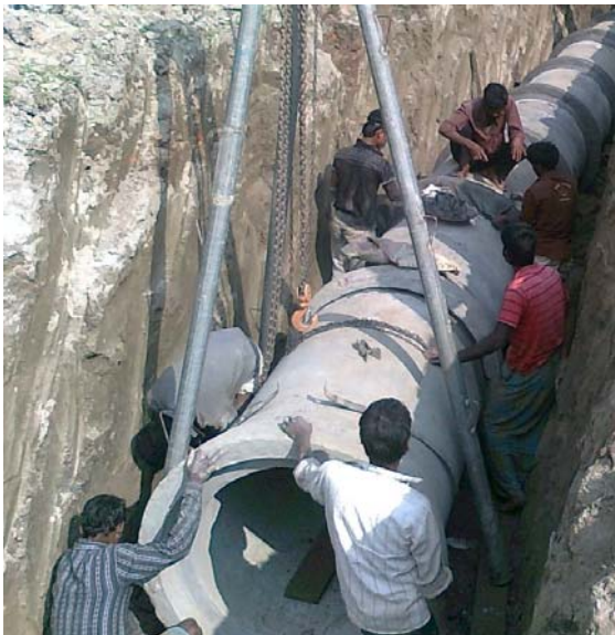
Placed concrete pipes with mortared joints SP 31001 Rouha, Mymensingh
