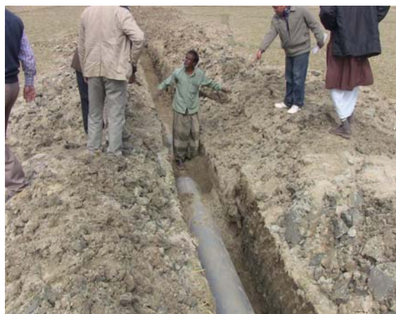
Backfill to uPVC Pipe SP 33097 Mongalpur, Sunamganj
