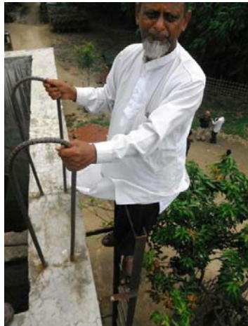
Access ladder arrangement to top of Header Tank, SP 25288 Dariapur, Chapai Nawabganj
