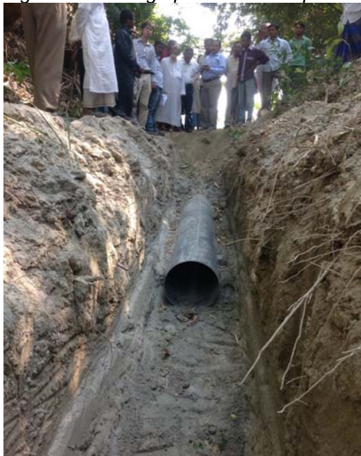
Figure I-1: Photographs of uPVC Pipe and T-fitting
