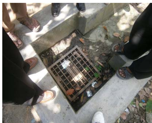
Locked cover to prevent tampering with alfalfa valve SP 25240 Chara Para, Unmesh, Mymensingh
