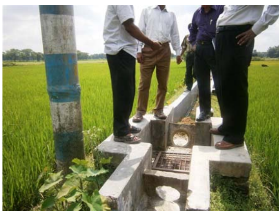
Outlet box arrangement with pucca-nucca to control flow to field channels SP 25240 Chara Para, Unmesh, Mymensingh
