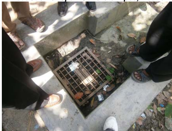
Locked cover to prevent tampering to Alfalfa Vale of Outlet
