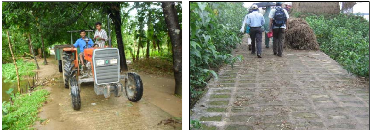
Figure 4.13: Rigid and block pavements
