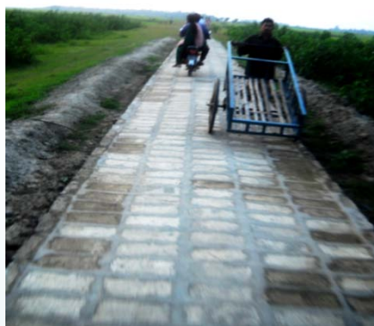
Newly built concrete block based submergible village road at Jamalganj, Sunamganj. For the first-time concrete block based village road introduced by CBRP-LGED. A total of 172 km block road has been built at different upazilas of Sunamganj for linking the remote villages with main road network and resource bases. The concert block road is highly flexibly to fit in with the flooding nature of Sunamganj and reasonably cost effective
